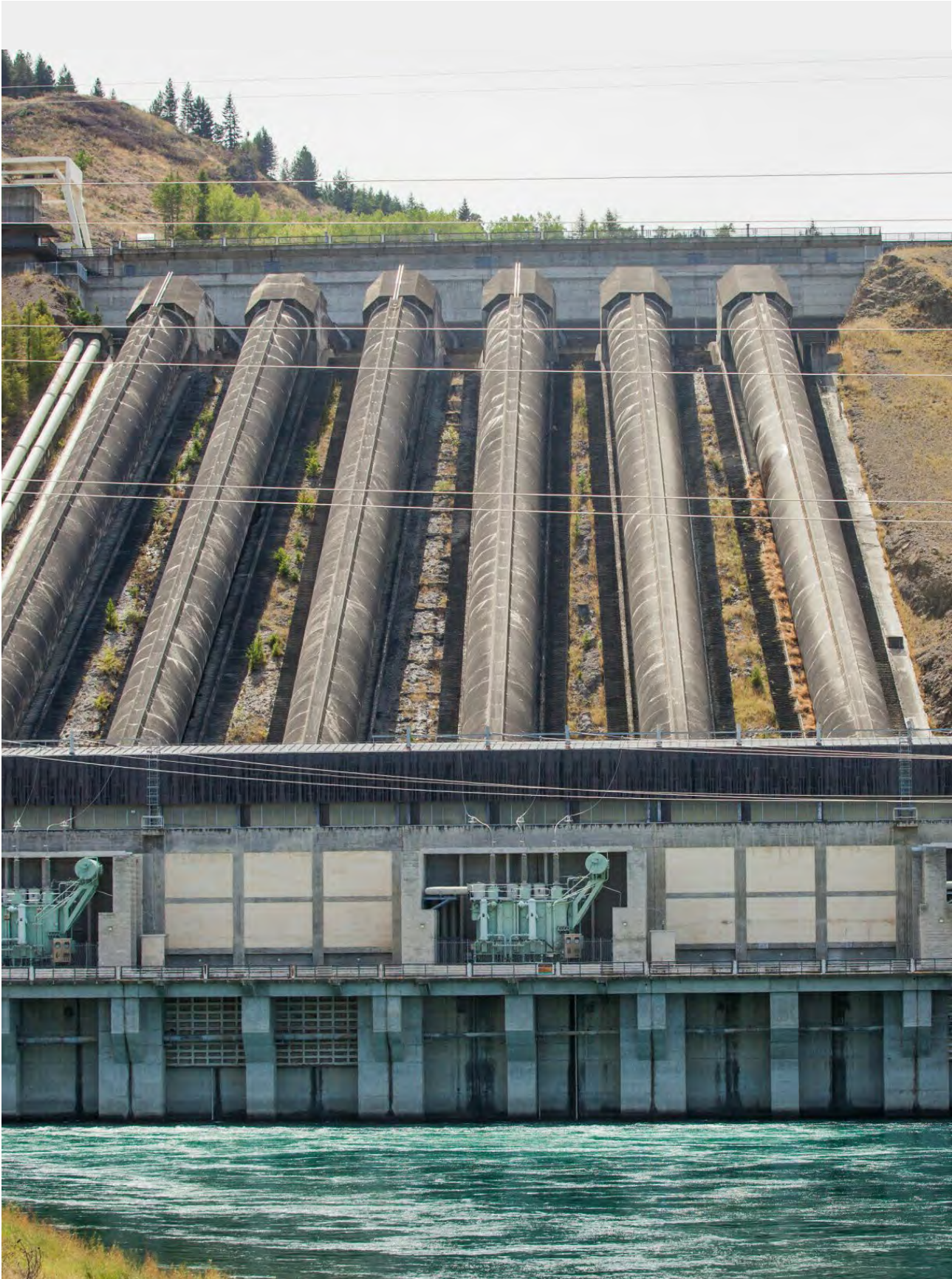
Hydro Dam, Lake Benmore, Canterbury. Credit: Kathryn Taylor, Truestock.
